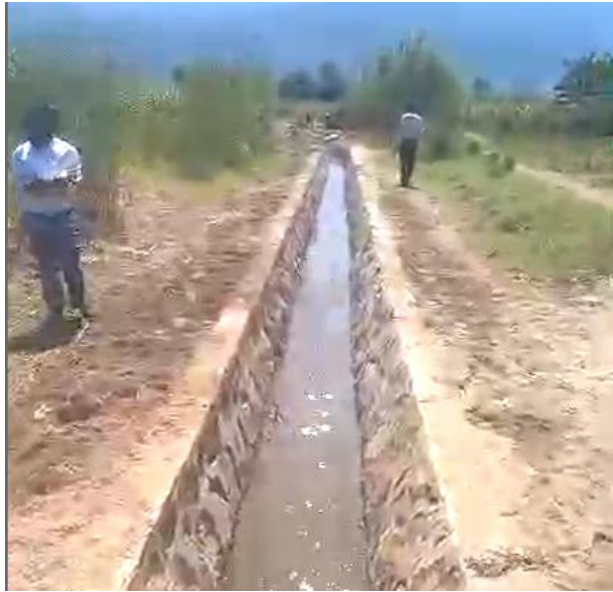
Plate 16: Iziwasungu Irrigation Canal at Iziwasungu Village, Mpimbwe DC
