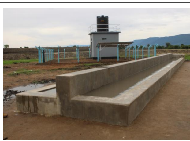
Plate 21: Water reservoir tank and cattle trough at Iziwasungu Village, Mpimbwe DC.
