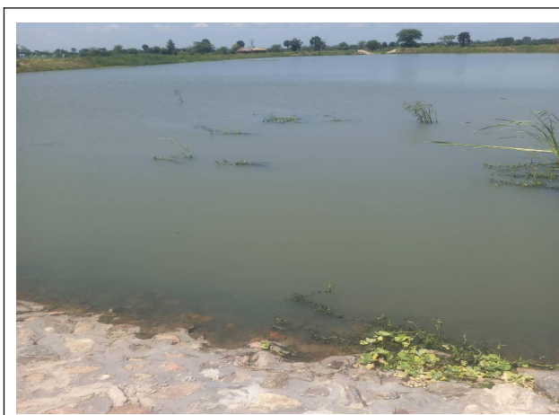
Plate 20: Charco dam at Iziwasungu Village, Mpimbwe DC
