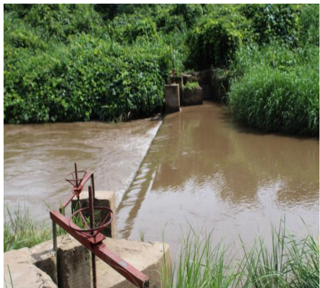
Plate 22: Water gates(3) in Katuma River, Mnyagala Village, Tanganyika DC
