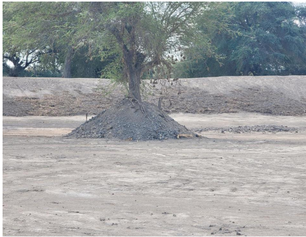
Plate 5: Construction of Charco dam at Idenyimembe Village, Wanging'ombe DC
