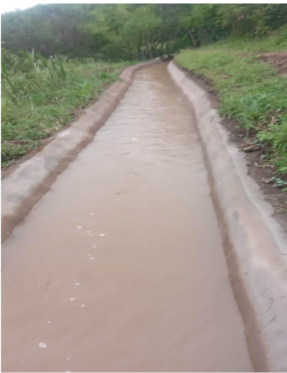
Plate 2: Rehabilitated irrigation canal of Ipwasi Ndorobo irrigation scheme, Kipera Village, Iringa DC
