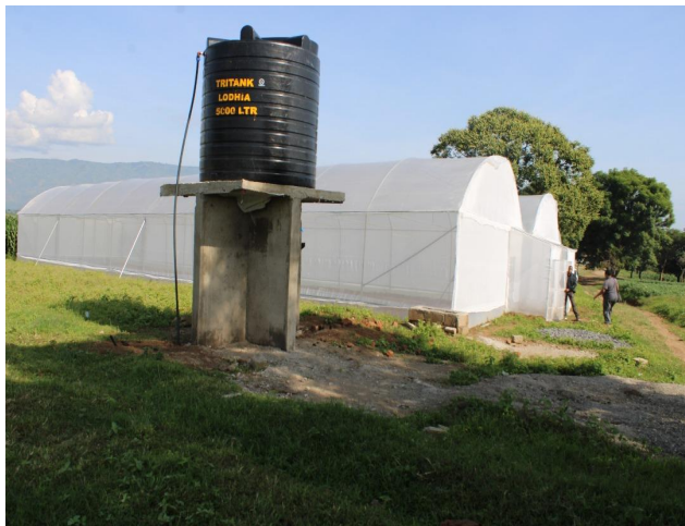
Plate 13: Two (2) screen houses for production of horticultural crops at Itewe Village, Mbeya DC
